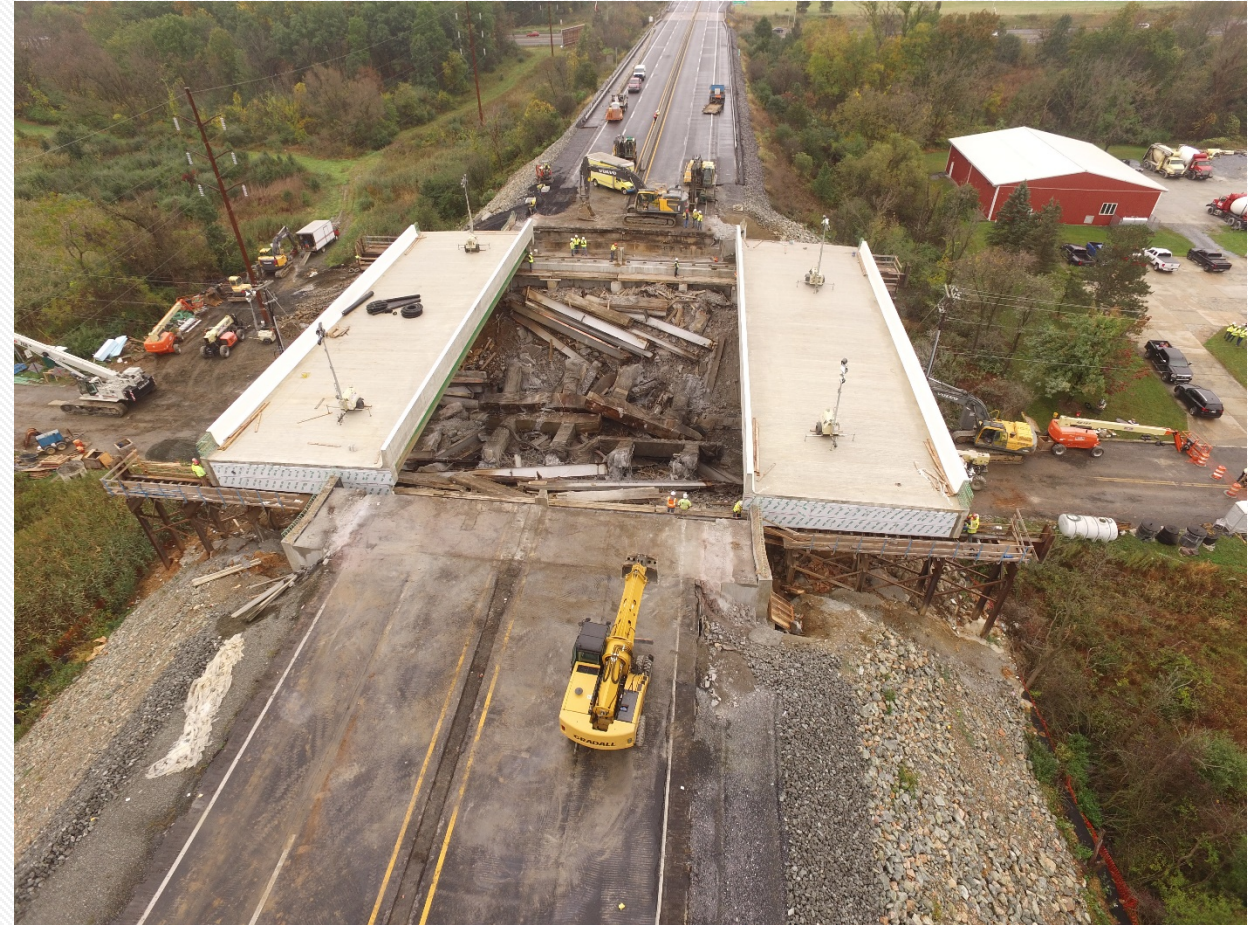
Accelerated Bridge Construction (ABC) at A57.66
